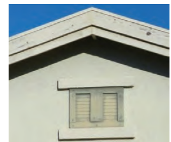
Wood Fascia and Architectural Feature
