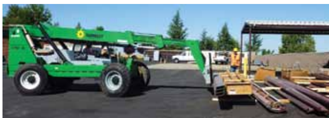
Metal components for the new Maintenance Building were delivered August 22
