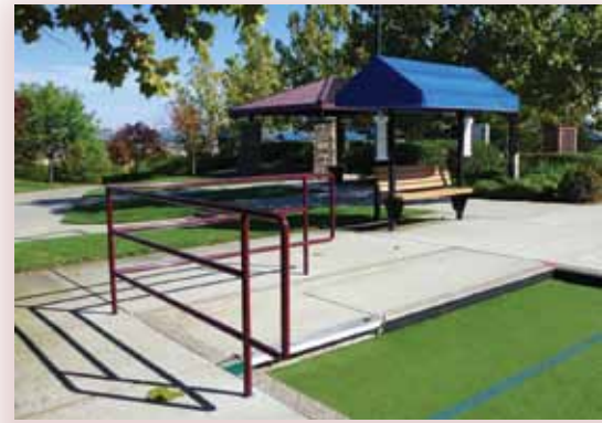
Small but important project: Safety railings installed at ramp trip hazard on Bocce Court #1
