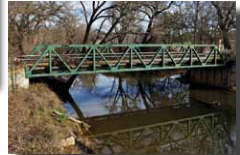
Old bridge at Coon Creek
