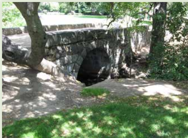
One of twelve granite bridges
