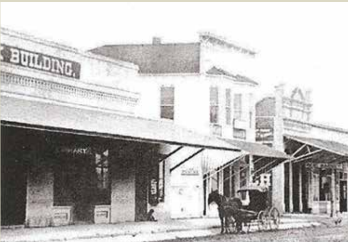
The New Fleming Building today (top) and in 1910
