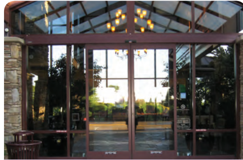
OCL Main Entry, New Doors
